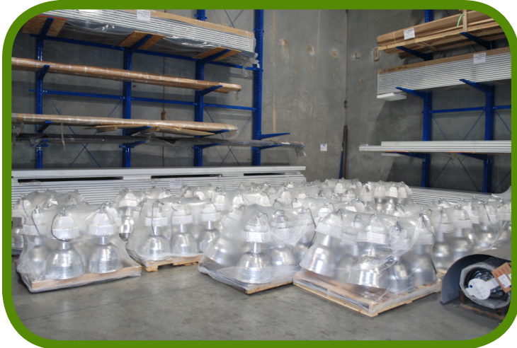
Removed High Bay Metal Halides & T12 Lights
